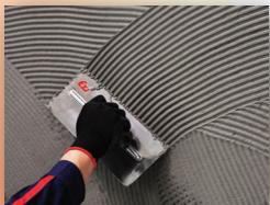
Spread paste on the substrate
