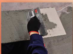
Spread paste on the back of tile
