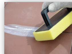
Applying the Grout
