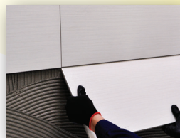
Place tile onto the adhesive bed
