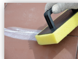
Applying the Grout
