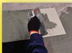
Spread paste on the back of tile
