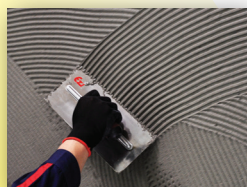
Spread paste on the substrate
