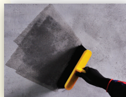
Make sure the surface is clean
