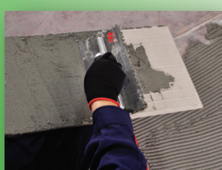
Spread paste on the back of tile
