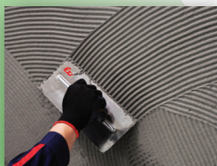
Spread paste on the substrate
