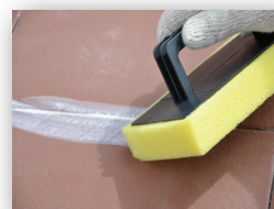
Applying the Grout
