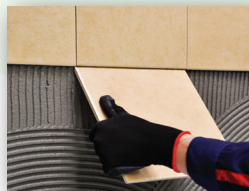
Place tile on the adhesive bed
