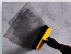
Make sure the surface is clean
