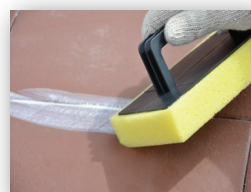
Applying the Grout
