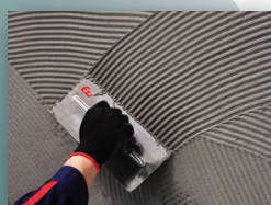
Spread paste on the substrate
