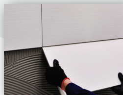
Place tile onto the adhesive bed
