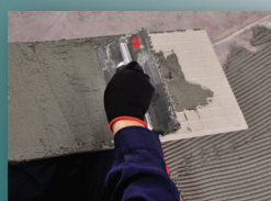
Spread paste on the back of tile
