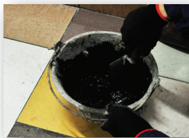
Mix Ezi GROUT FINE with clean water or latex admixture as per recommended ratio.
