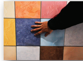
The wall grouting is completed
