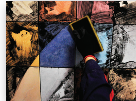
Clean & remove excessive grout immediately with damp cloth or sponge.
