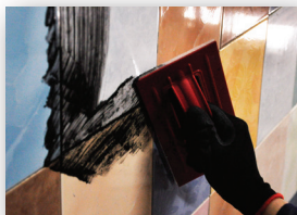
Spread grout to the joints with grout float or rubber squeegee.
