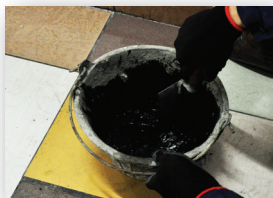
Mix Ezi GROUT COARSE with clean water or latex admixture as per recommended ratio.
