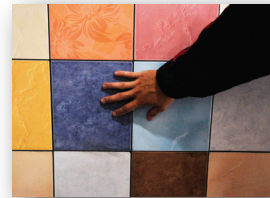
The wall grouting is completed
