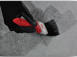
Apply Ezi H2O SEAL to the top surface of natural stones with a brush or roller.
