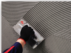
Spread paste on the substrate
