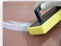
Applying the grout
