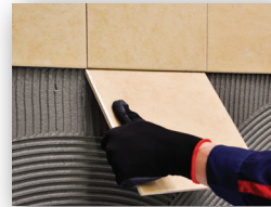
Place tile onto the adhesive bed
