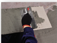
Spread paste on the back of tile
