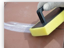
Applying the Grout
