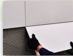
Place tile onto the adhesive bed
