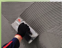
Spread paste on the substrate
