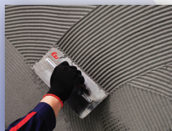
Spread paste on the substrate
