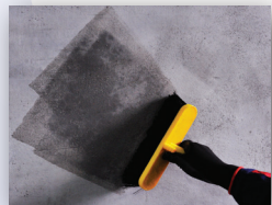
Make sure the surface is clean
