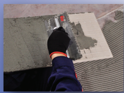
Spread paste on the back of tile
