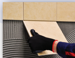
Place tile onto the adhesive bed
