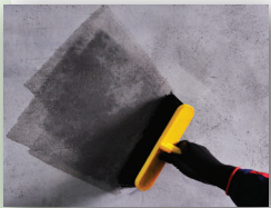
Make sure the surface is clean
