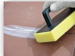
Applying the Grout
