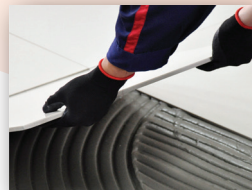
Place tile onto the adhesive bed
