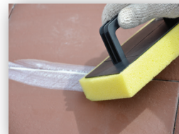
Applying the Grout
