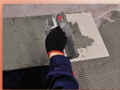
Spread paste on the back of tile
