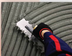
Spread paste on the substrate
