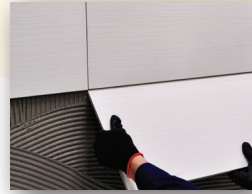
Place tile onto the adhesive bed
