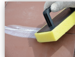
Applying the Grout
