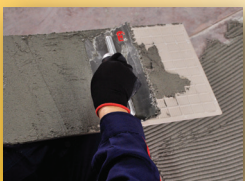
Spread paste on the back of tile
